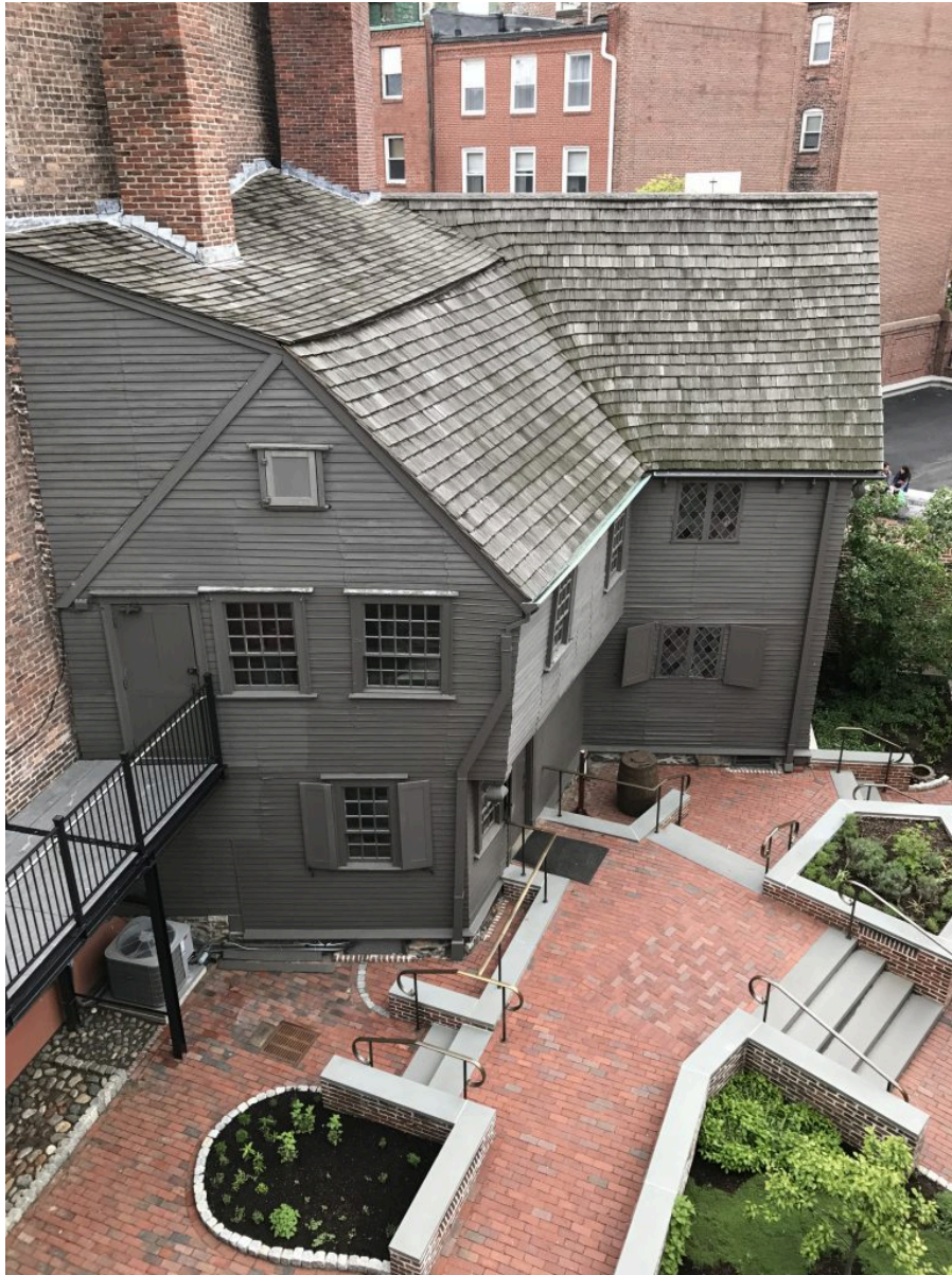
Paul Revere House, Boston, Massachusetts, as seen from Lathrop Place. Access to the first floor of the Paul Revere House for those in wheelchairs is through a ramped and widened doorway to an early kitchen addition, the same entrance used by all visitors to the site. Second-floor access is by a bridge from the neighboring Lathrop Place, an 1835 building that was rehabilitated with an elevator for visitor use. Photograph by Cynthia G. Falk, May 2017.
