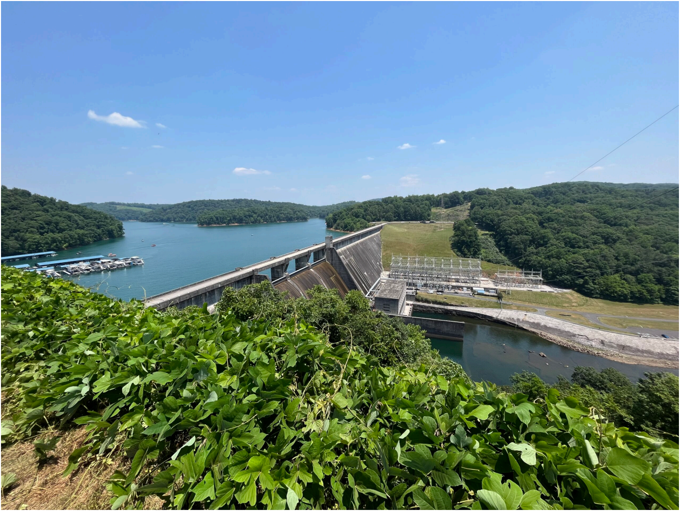
Norris Dam, Tennessee. Photo credit: Karen-Beth G. Scholthof
